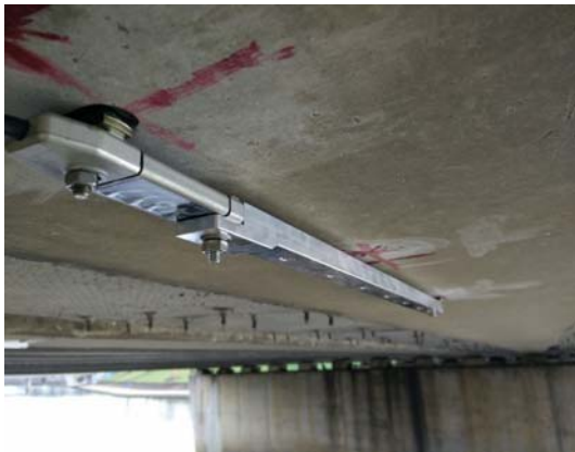
Figure 3: Strain Transducer attached on a girder soffit with aluminium extension rod.
