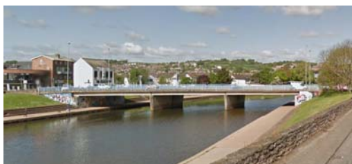
Figure 2: Exe North Bridge Spanning River Exe.
