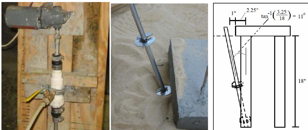
Fig. 14. Grout tube connected to grout swivel and subsequent installation
